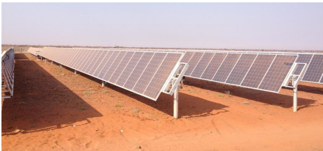
Figure 5-8: A single axis tracking system
